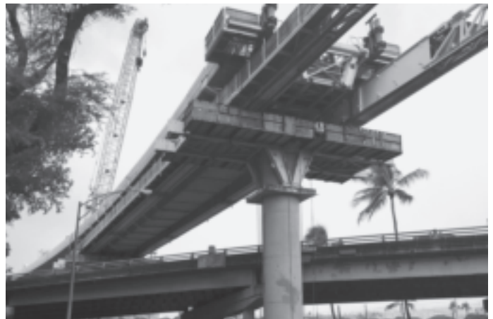
Constructing the rail guideway.
