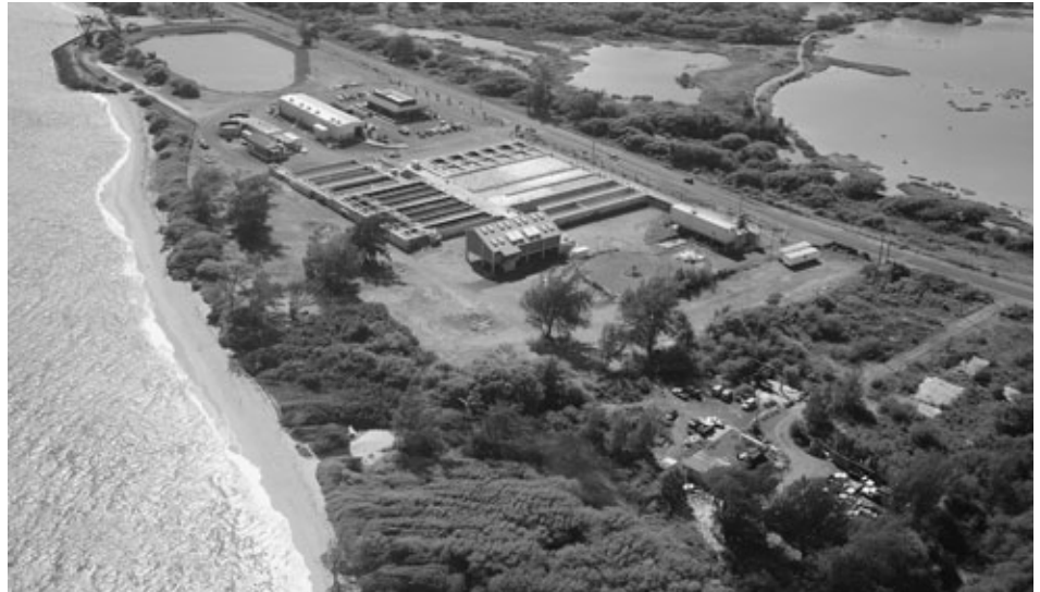
Wailuku-Kahalui Wastewater Facility Improvements Project for Maui County by Brown and Caldwell.
