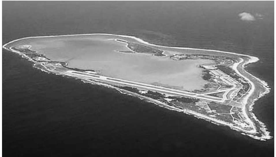
Military Construction program on Wake Island by Earth Tech, Inc.
