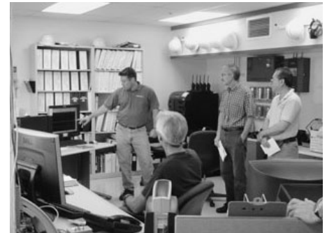
The simple Kapaia Power Station Control Room.
