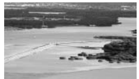
SSFM: Dredging for the Fort Kamehameha Wastewater Treatment Plant Outfall.
