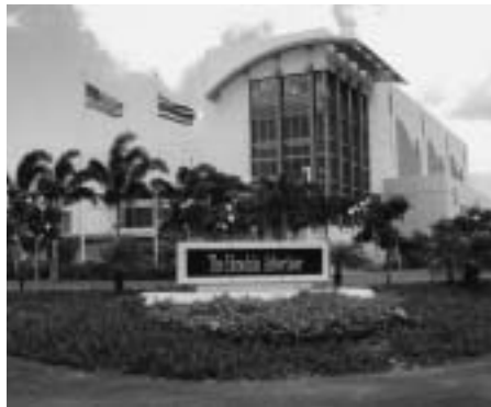
Notkin: Honolulu Advertiser Production and Distribution Facility with Displacement Air Type System.
