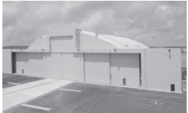
OCEA Award Winning Project: Design-Build AEF FOL Aircraft Maintenance Hangar, Andersen Air Force Base, Guam.
