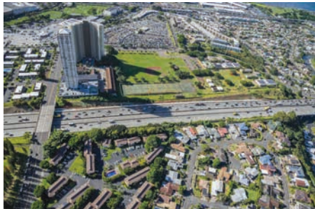
Excellence Award, Post Construction Photo of the Completed Interstate H-1 Shoulder Work and PCC Rehabilitation
