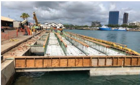
Honor Award, Installation of Precast/Prestress Concrete Slab Sections in Progress
