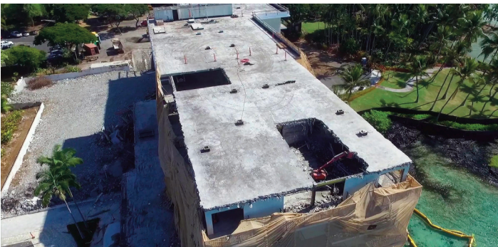
Excellence Award: Aerial Photo of Above Water Demolition
