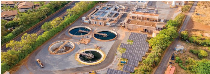
Excellence Award: Lahaina Waste Water Reclamation Facility Aerial View
