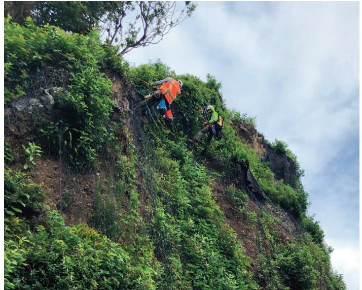
Checking rock bolts along slope on completed project.
